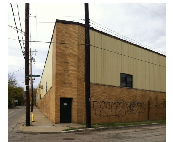
Warehouses located along Elmore St and Dreman Ave
